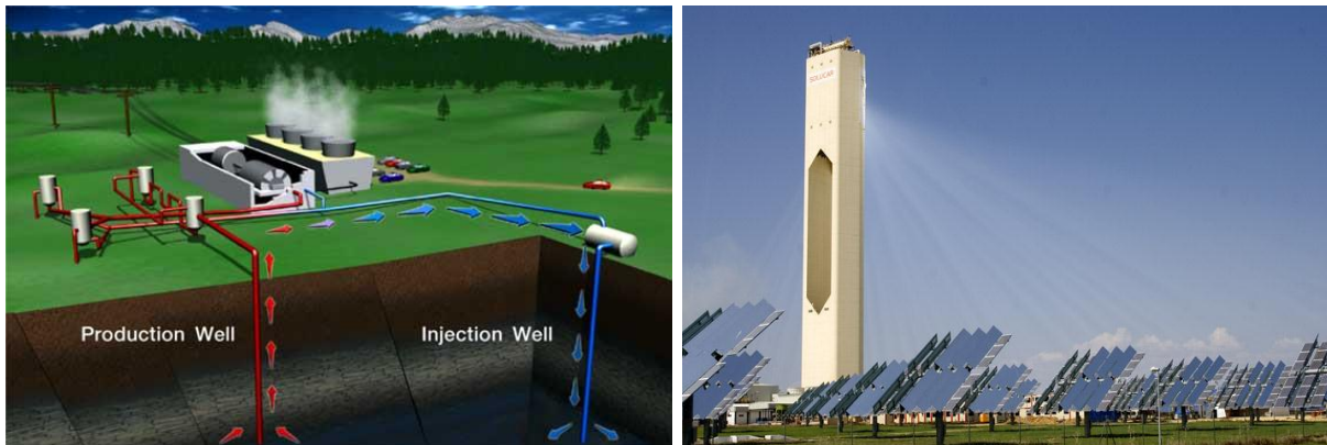
Figure 9: Left: artist impression of a geothermal electric powerplant (taken from energy-green.net); Right: concentrated solar electric plant Solúcar PS10 (taken from Wikipedia)
