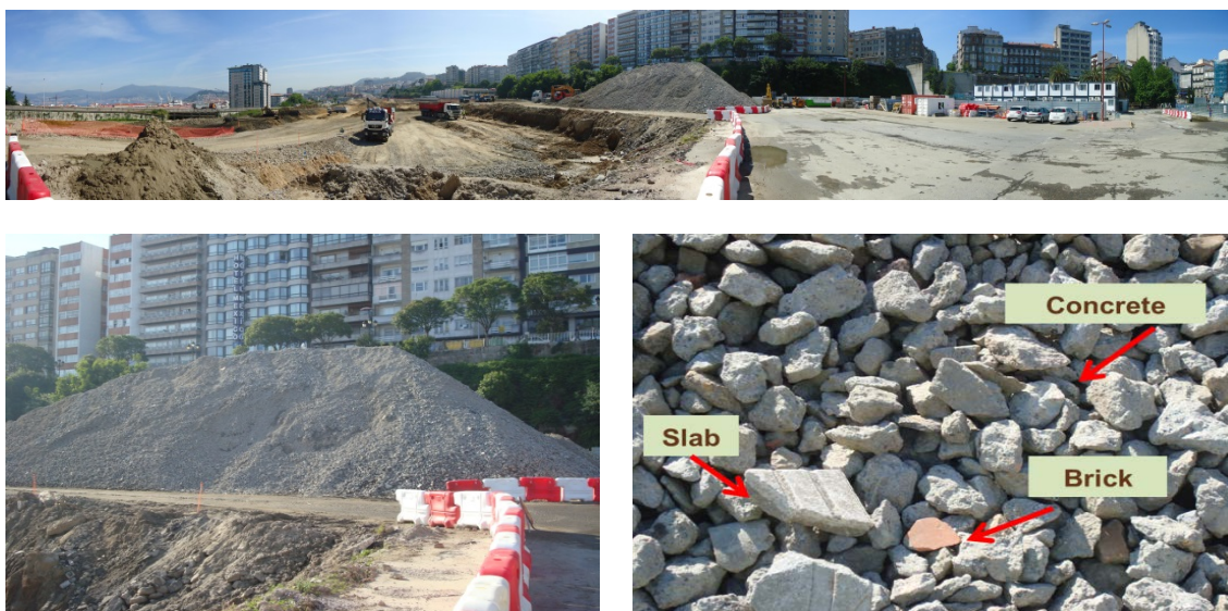
Figure 26: Stony fraction recovered from the demolition works
