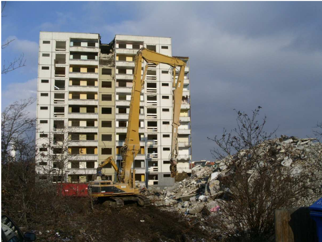
Figure 7: Demolition of prefabricated housing estates in Halle, Germany.
