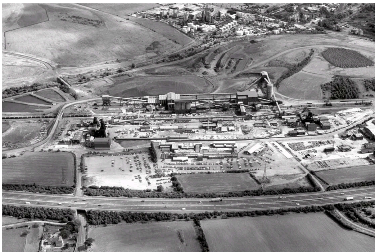
Figure 14: Former colliery site adjacent to the M1.
