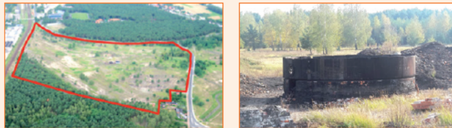
View of the case study site in Solec Kujawski (left) and view on parts of the brownfield site with half full creosote container (right)
