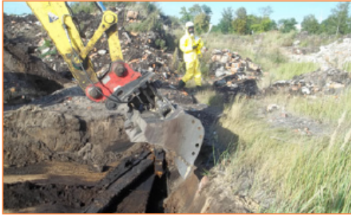
Figure 3: Contaminated underground Installation found during excavation works (done during the preparation for the soil washing field tests within the TIMBRE project) (Photo: Geo-Logik)
