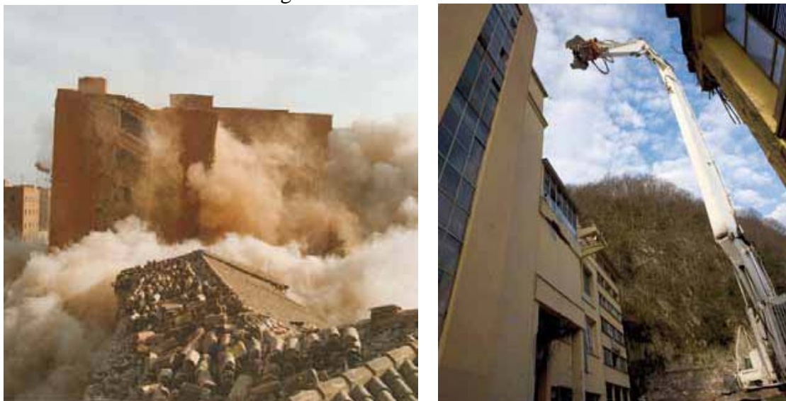
Figure 9: Intensive demolition: explosive demolition (left) and long arm reach for mechanical demolition (right). Source: www.aeded.org
