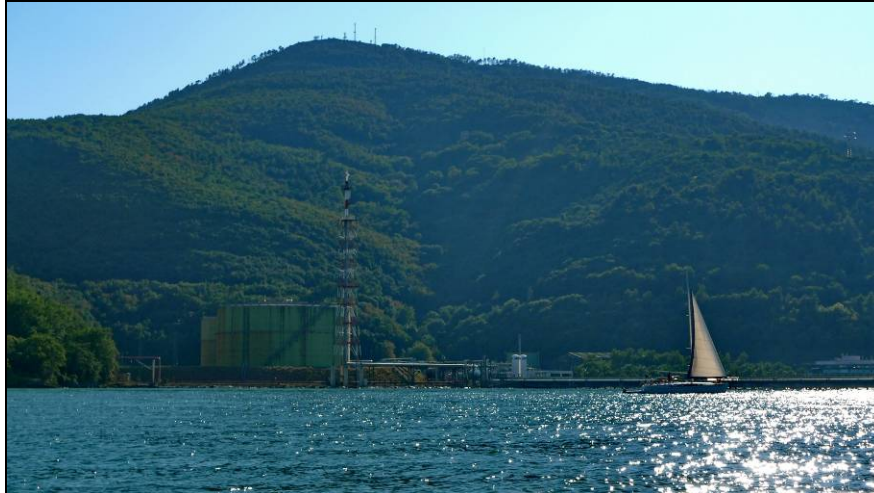
Figure 12: ENI LNG Terminal of Panigaglia in La Spezia Gulf, Italy
